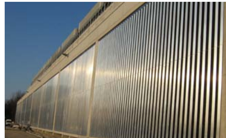
Splitter silencers for cooling towers; GEA Energietechnik GmbH, project Mellach, Austria
