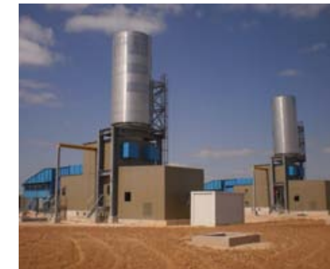
Acoustic Enclosure for THM Gas Turbine; MAN Diesel & Turbo SE, project Villarpipe, Spain
