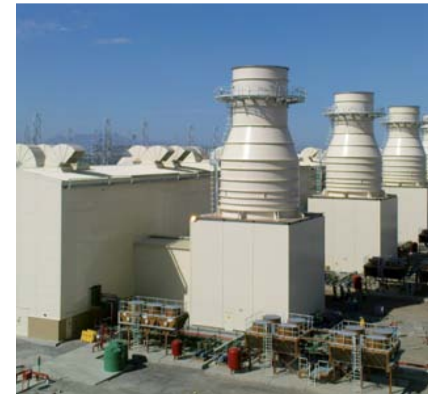
Left: Outdoor noise enclosure for gas turbine GT 13; Alstom AG, project Colongra, Australia Right: Noise and weather enclosure for gas turbines; Roshcon, project Ankerlig
