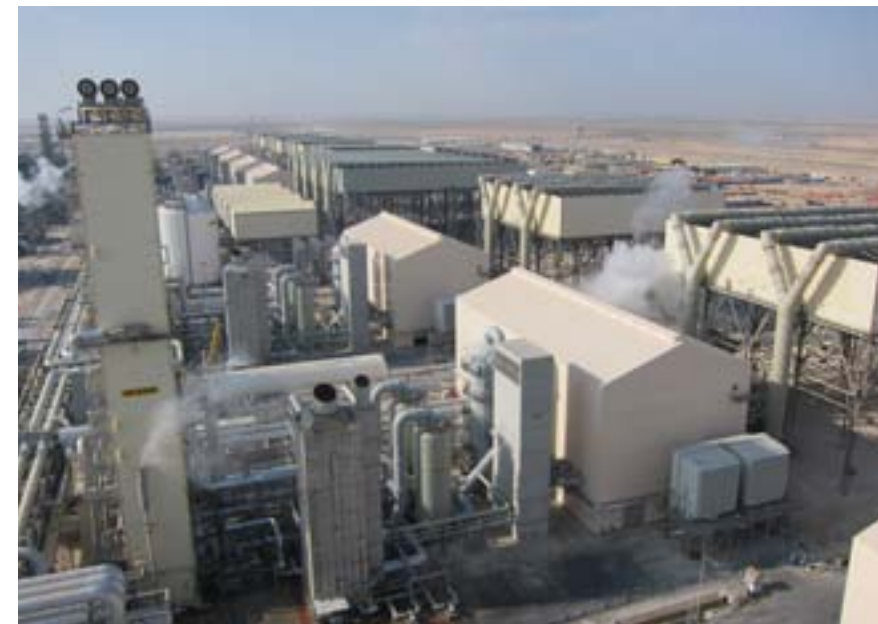
Below: Noise enclosure for compressors, Gas-to-Liquid-Plant; Linde AG; project Pearl Qatar
