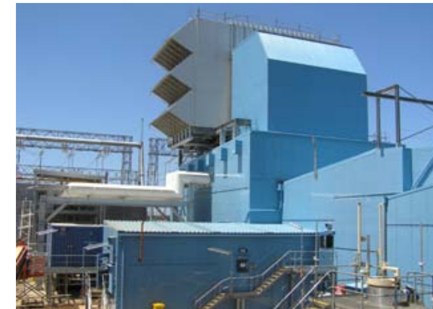
Above: Air Intake with weather hoods and multi stage filter (combi filter) Left: Noise enclosure for gas and steam turbines, Siemens AG, project Sloe Centrale, NL Right: Noise enclosure for open cycle power plant, SGT5-4000F, Siemens AG, project Mortlake, Australia
