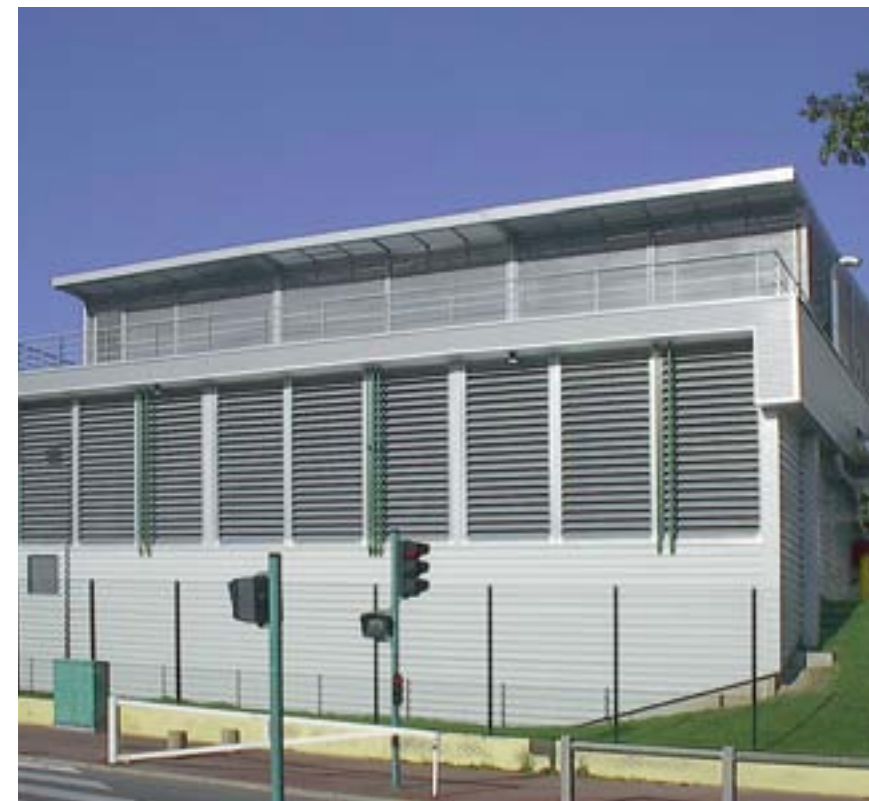
General noise concept for cogeneration plant; Wärtsilä Power Plants; project Aulnay-sous-Bois, France
