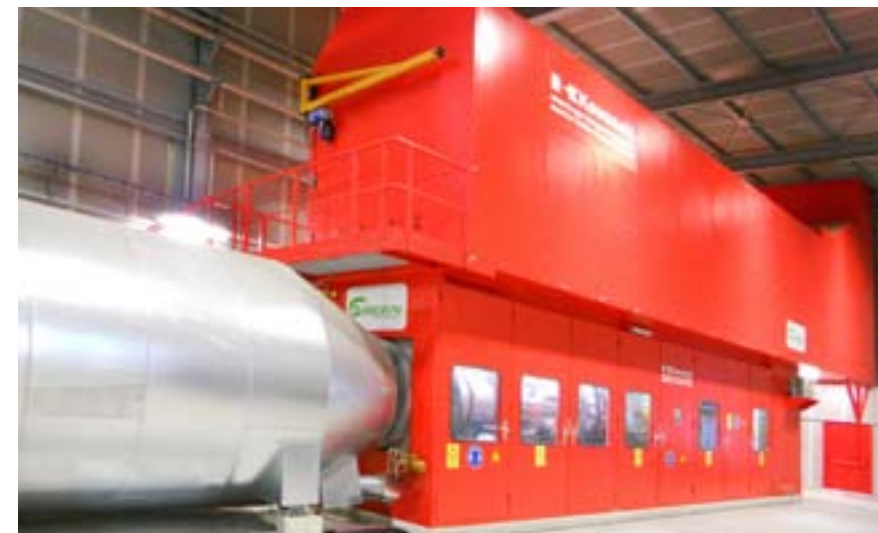
Below: Noise enclosure for compressors, Gas-to-Liquid-Plant; Linde AG; project Pearl Qatar
