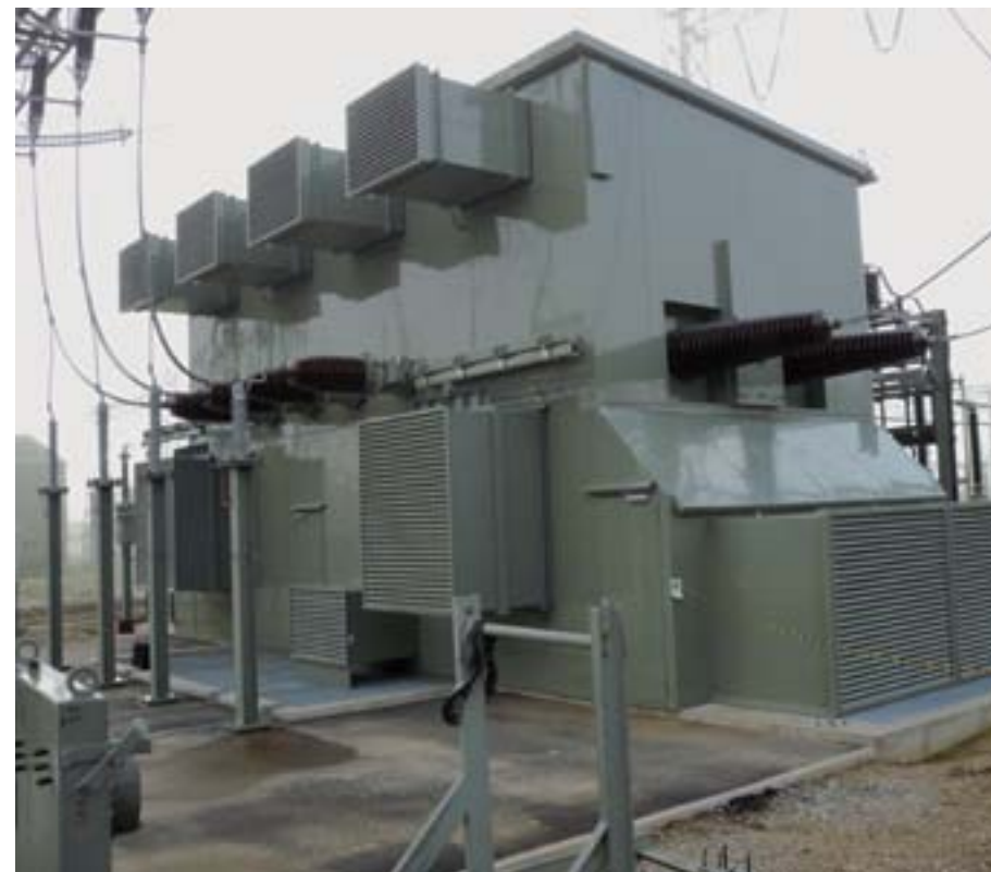
Above: Sound enclosure for transformer station, project E.ON, Germany Left: Noise enclosure and filter house for gas turbine generator set GPB 80 of KAWASAKI Gas Turbine Europe Right: Air flow concept of GT compact package unit MAN Diesel & Turbo SE
